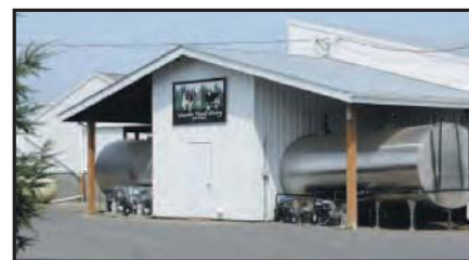
Vander Haak Dairy's milking facility is 1.5 miles away from the heifer and dry cow barns and digester.
